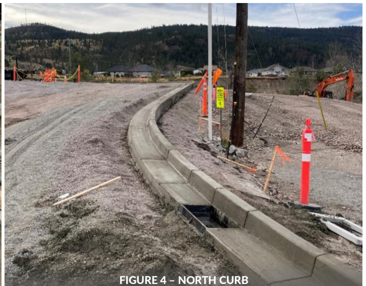
FIGURE 2 – CATCH BASIN INSTALL
