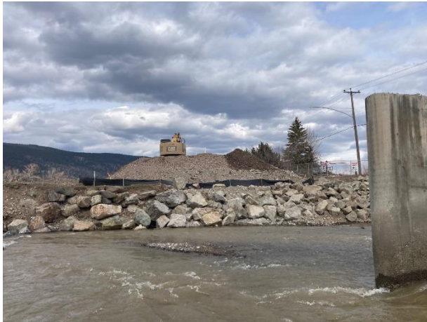
Figure 1 - Pre-load at the North Abutment
