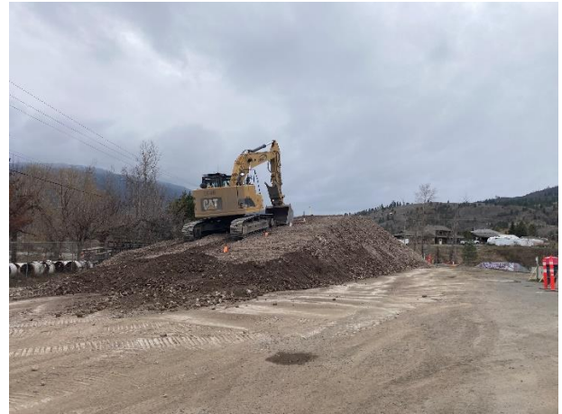
Figure 2 - Pre-Load at the north abutment and settlement gauges
