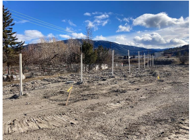
Figure 2 – Survey, layout and install preload gauges
