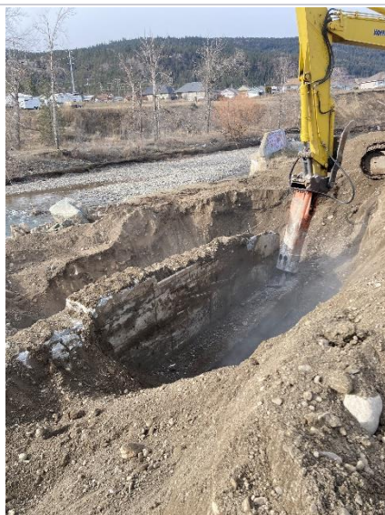
Figure 3 – Demolition of remainder of north abutment
