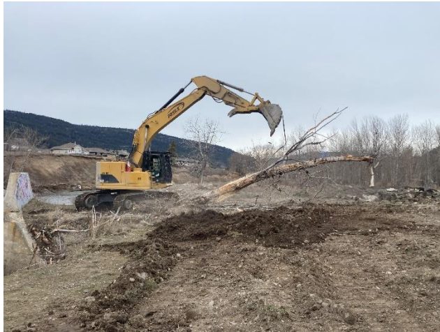
Figure 1 – Removal of northwest tree which overhung the river
