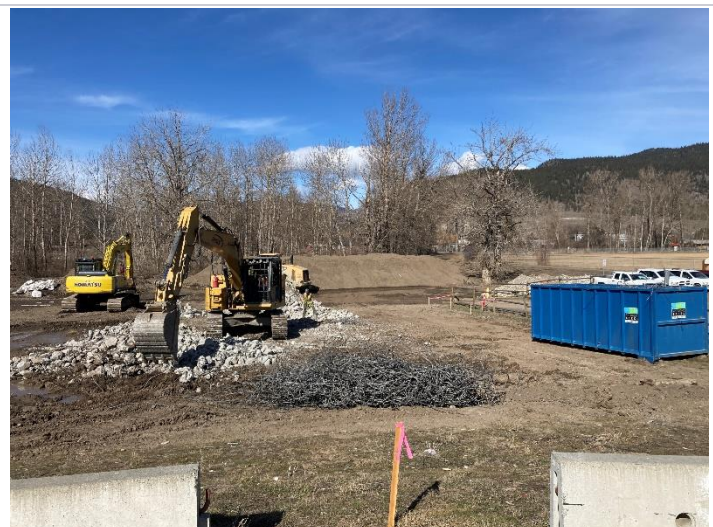
Figure 4 – Processing demolition materials, spreading rebar from concrete
