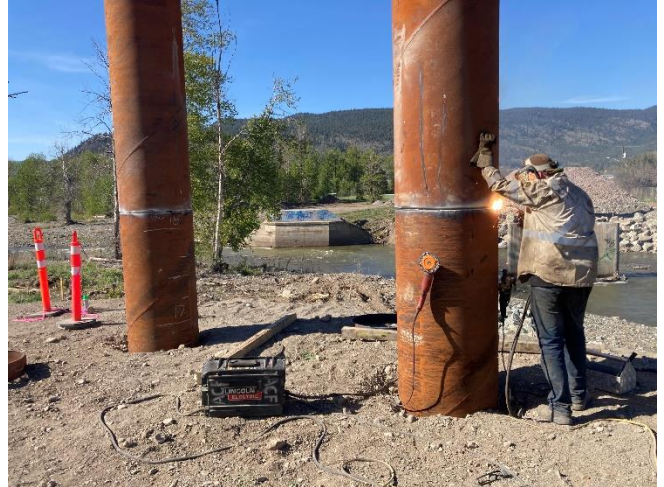
Figure 2 – Welding pile splice
