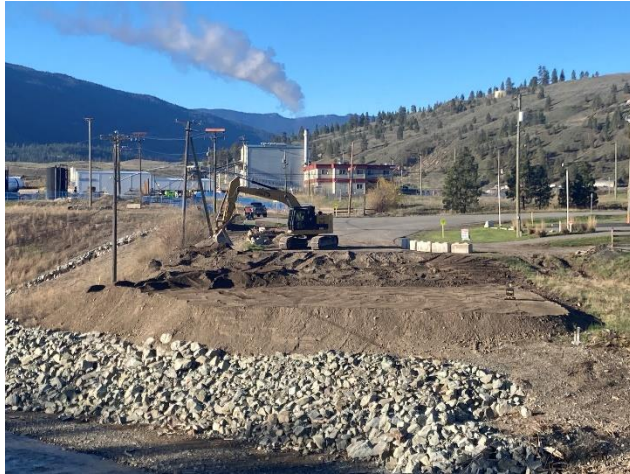
Figure 1 – Construction of south crane pad
