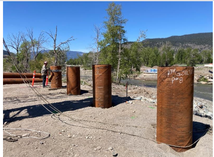
Figure 4 – South Abutment pile driving
