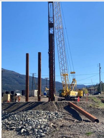
Figure 3 – South Abutment pile driving
