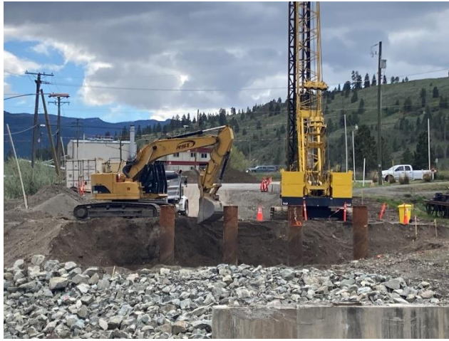
Figure 1 – Excavating to pile cut off
