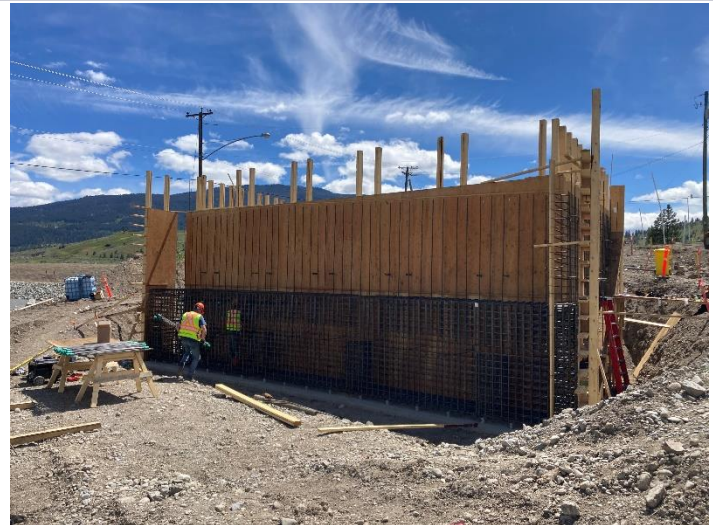
Figure 4 – South Abutment reinforcing steel
