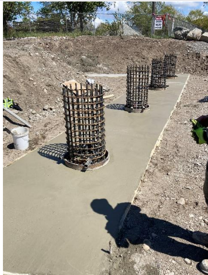
Figure 3 – North Abutment mud slab
