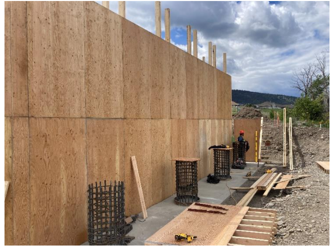
Figure 2 – South Abutment formwork
